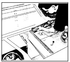
Seal joints along pipe chase seam with the caulk provided.
