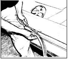
Insert nose bumper into master bumper channel. Roll nose bumper into channel along entire lineup (up to 96'). We recommend that the nose bumper be left in the store 24 hours before installing. DO NOT STRETCH the bumper during installation as it will shrink to its original length and leave a gap.
