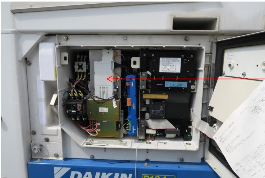
RMM-W mounted on isolated plate
