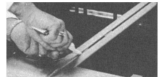
FIG. 4: Applying silicone
