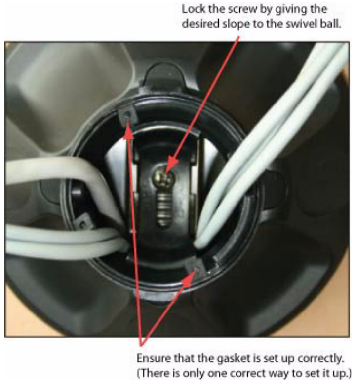
Figure 17 Routing the cables into the swivel
