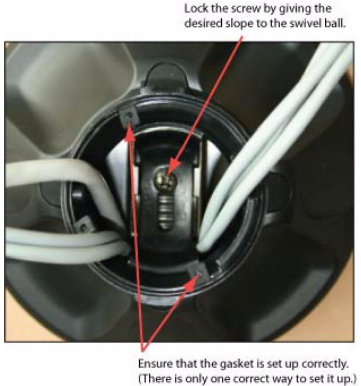
Figure 17 Routing the cables into the swivel
