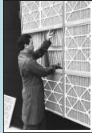
Installing filters and prefilters
