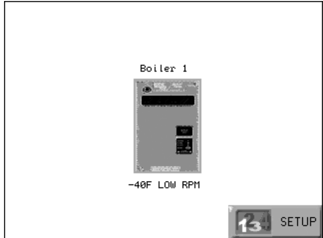
Fig. 6. S7999B Home page (Boiler 1 in normal operation).
