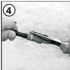
5. Connect the new drain hose to the waste Water pipe.
