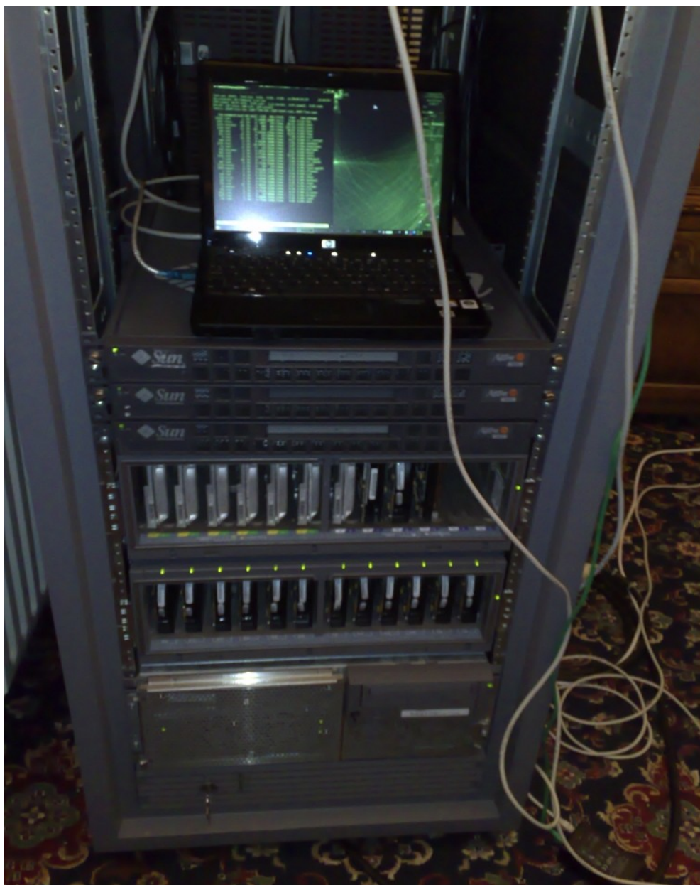
Img-5. Hp 2230s Data Center performance.
