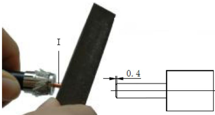
**Step 8** Use a brush to remove impurities from the cross section of the feeder, as shown in [Figure 5-104](#).
