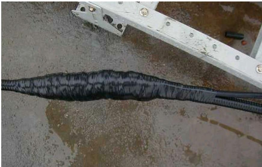
**Figure D-4** Wrapping lightning protection grounding clip with three layers of tapes
