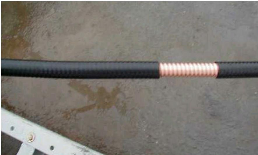
**Figure D-2** Striping off feeder skin
