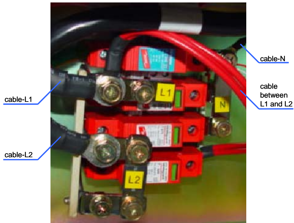
Figure 5-44 Connecting the 110 V power cables
