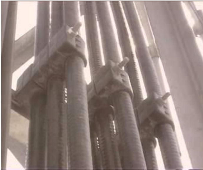
Figure 6-60 Fixing the feeders on the tower (using the 1-for-3 fixing clip)
