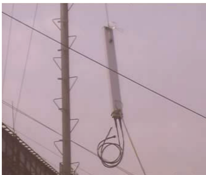
Figure 6-25 Hoisting the directional antenna
