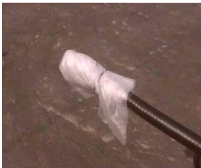
Figure 6-5 Simple protection of a feeder connector
