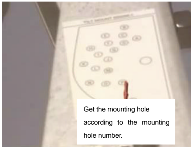
Figure 6-34 Directional antenna with the mounting hole corresponding to the pitch angle
