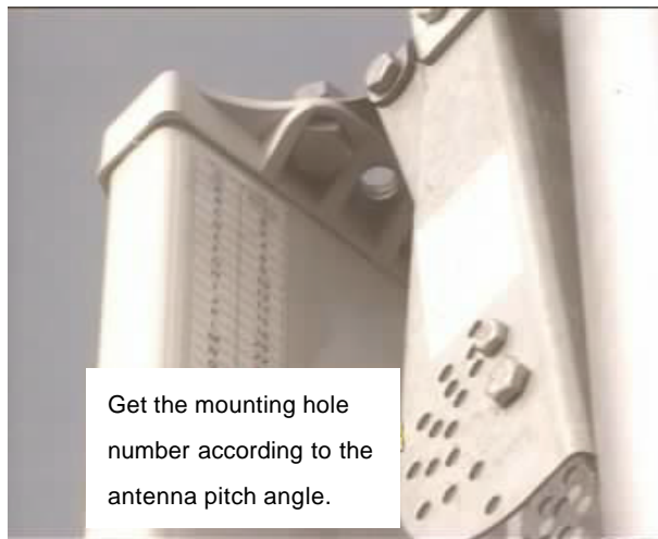
Figure 6-33 Directional antenna with the mounting hole corresponding to the pitch angle
