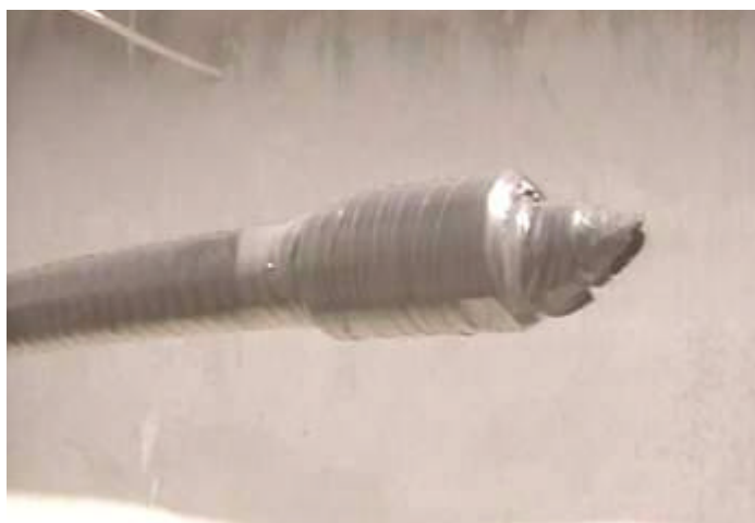
Figure 6-6 Simple waterproof treatment of a connector
