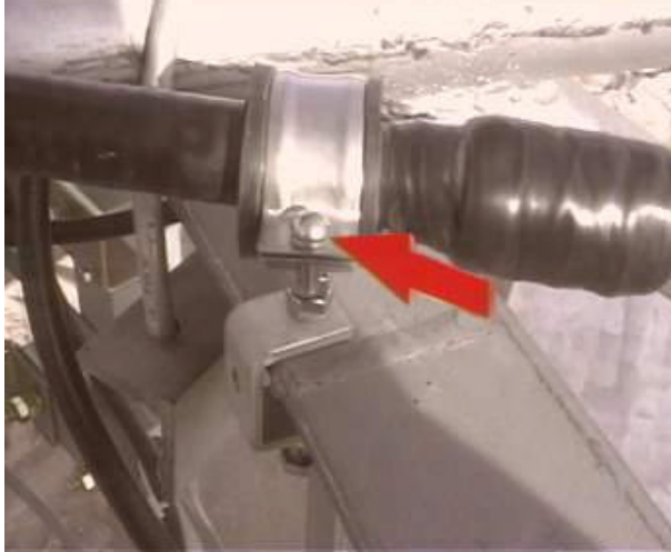
Figure 6-54 Fixing the upper end of the feeder on the tower
