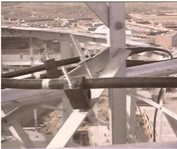
Figure 6-61 Fixing the feeders on the tower (using the 1-for-2 fixing clip)
