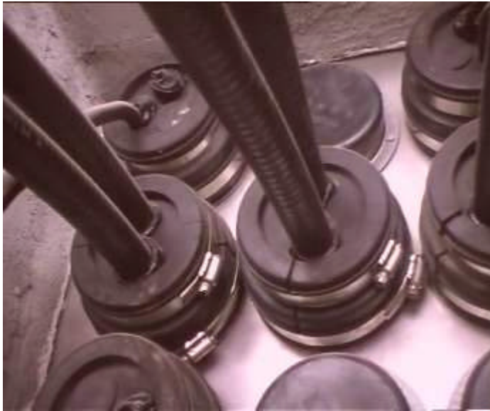
Figure 6-75 Feeder encapsulated window applied with waterproof & encapsulation treatment
