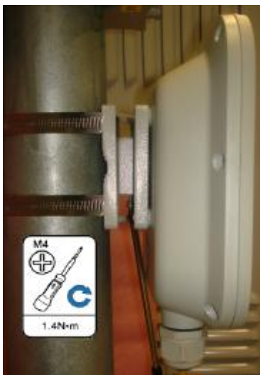
Figure 3-7 Tightening the screw
