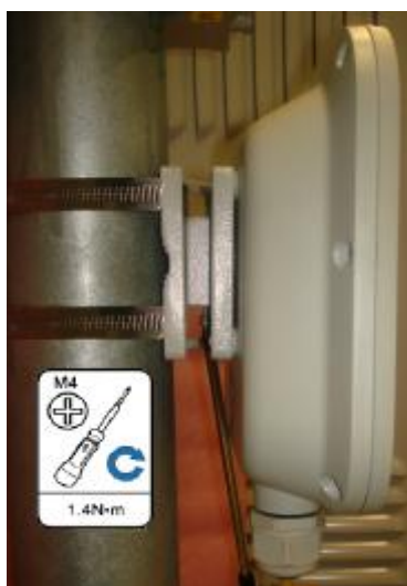
Figure 3-7 Tightening the screw
