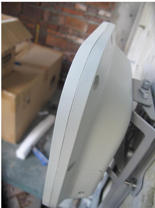
Figure 3-12 Fixing the LTE CPE
