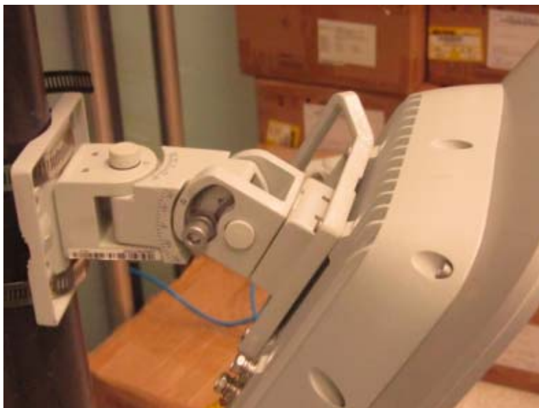
Figure 3-19 Installing the eA660 on the angle adjusting component
