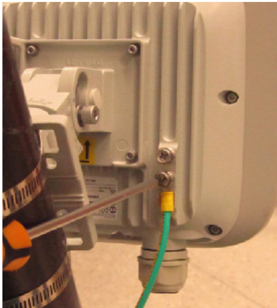
Figure 3-38 Connecting the ground cable
