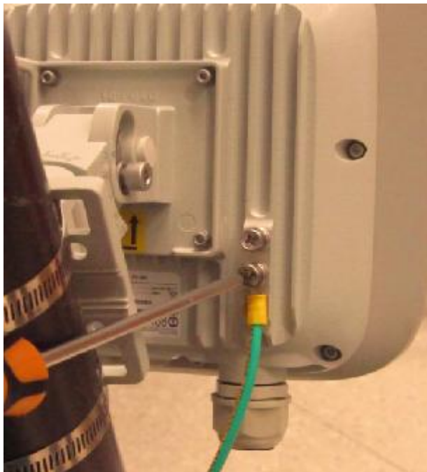
Figure 3-17 Connecting the ground cable
