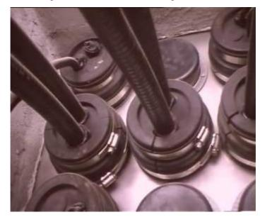
Figure 3-38 Encapsulation treatment of the feeder window after feeder enters the equipment room
