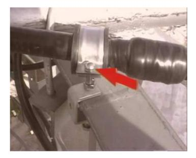
Figure 3-35 Feeder upper end fixed on tower
