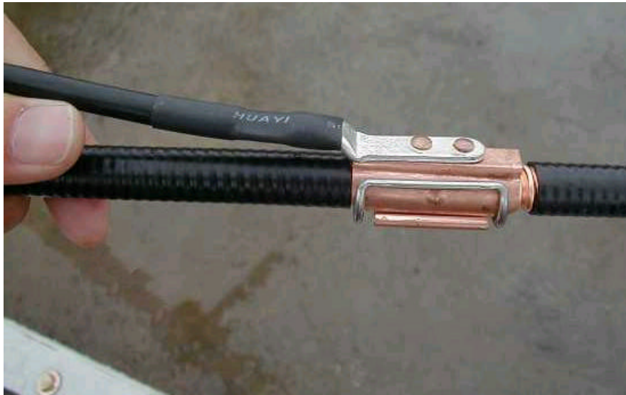
Figure D-3 Lightning protection grounding clip fixed on feeder
