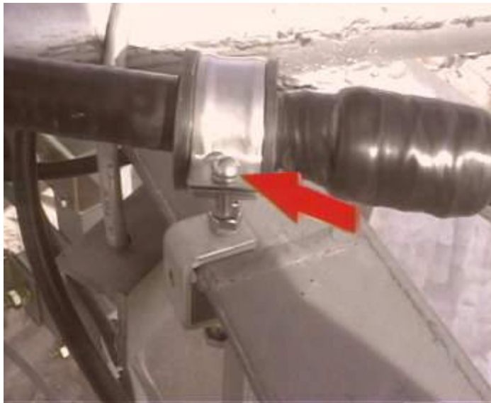
Figure 3-35 Feeder upper end fixed on tower
