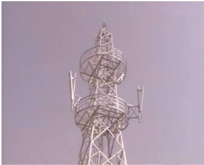
Figure 3-25 Installing the directional antenna on the tower side
