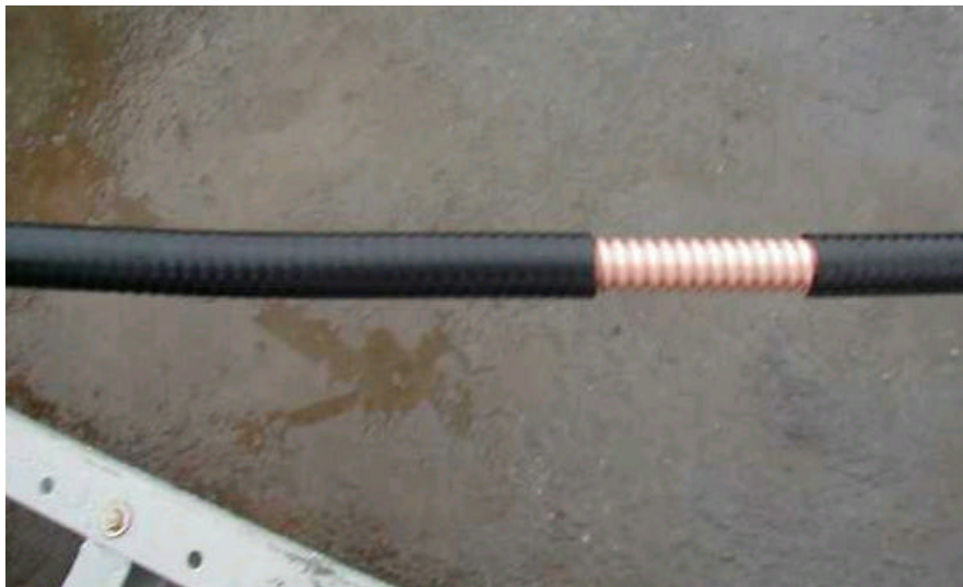
Figure D-2 Striping off feeder skin
