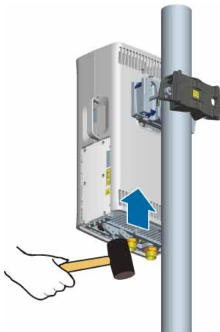
Figure 2-4 Knocking the RRU3606
