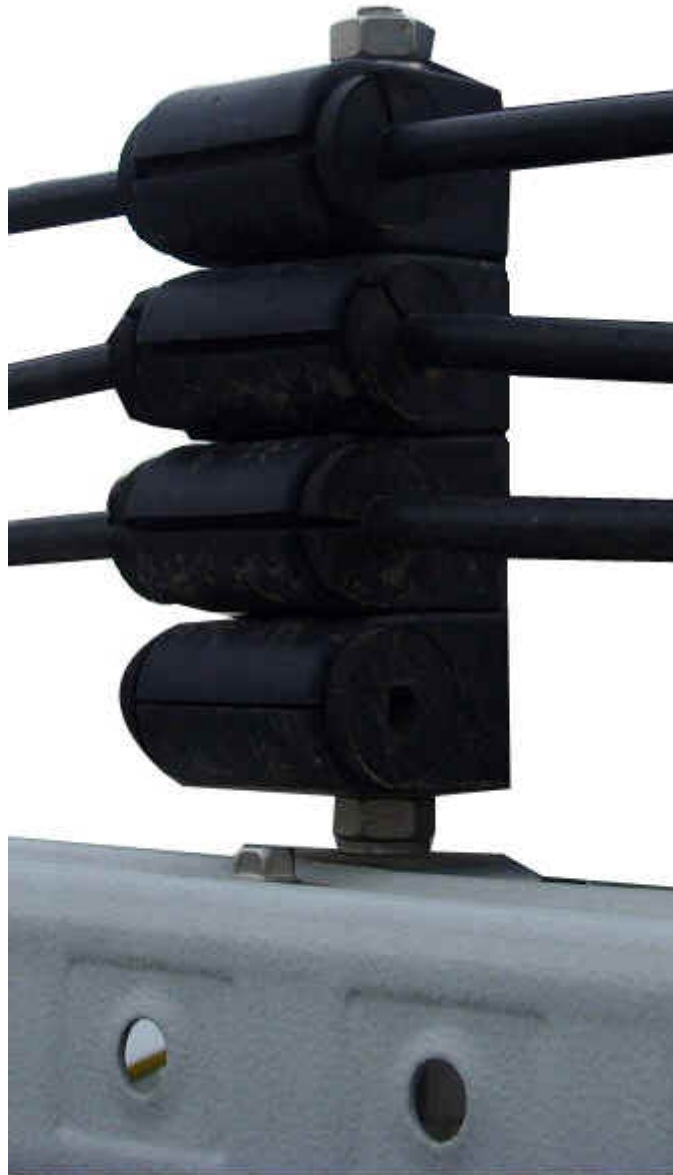
Figure 3-14 Installing the cable clip
