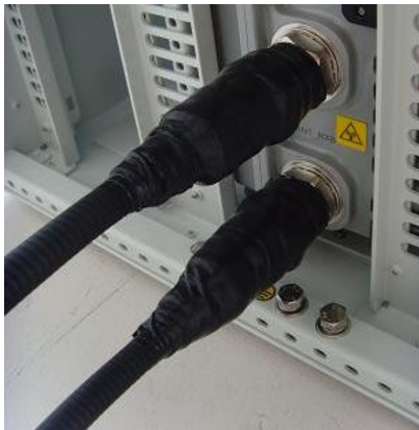
Figure 3-116 Waterproofed joints
