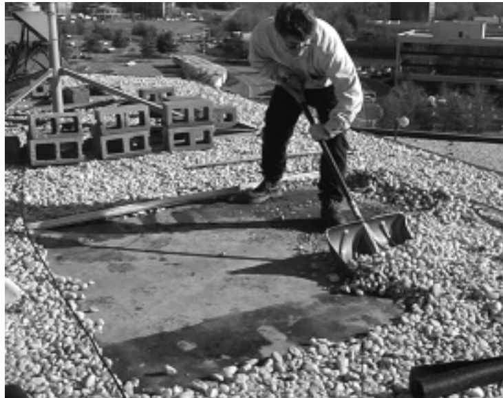
Figure 3-3 Clearing gravel from the installation location
