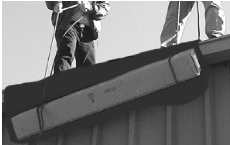
Figure 3-2 Hoisting materials to the installation location
