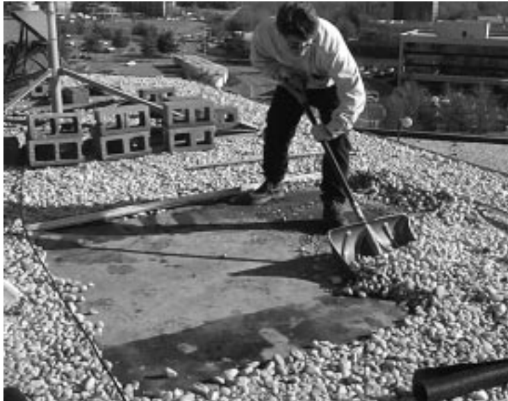
Figure 5-2 Clearing gravel from the installation location
