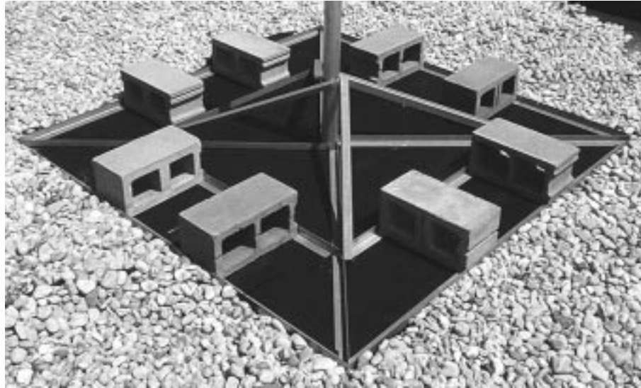
Figure 3-9 Proper placement of concrete blocks on the mount
