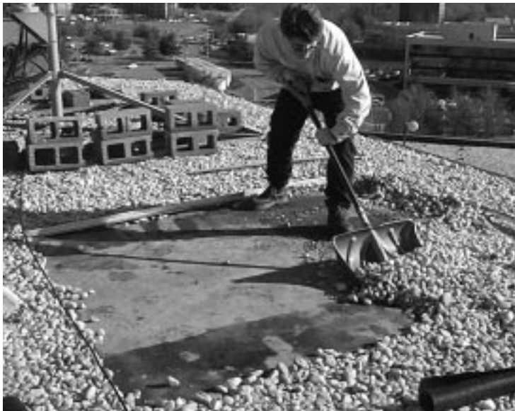
Figure 3-3 Clearing gravel from the installation location
