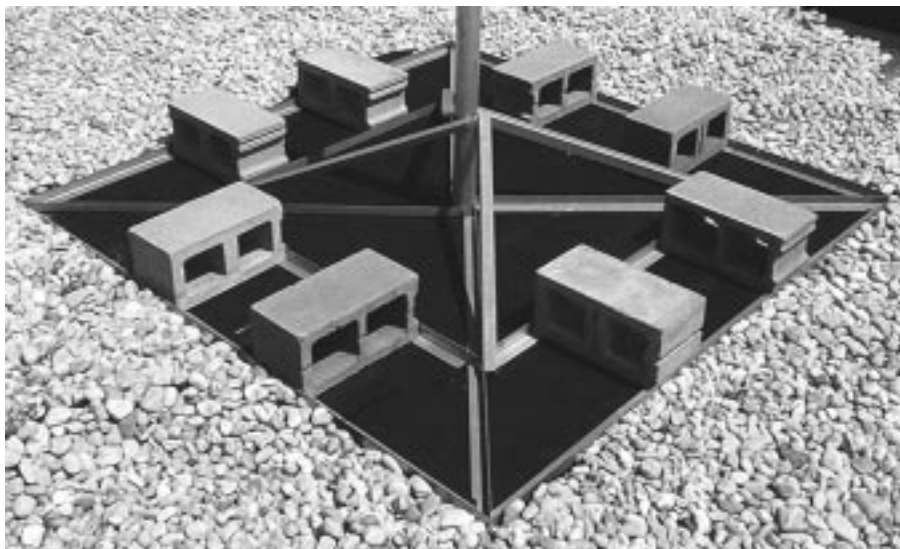
Figure 5-8 Proper placement of concrete blocks on the mount
