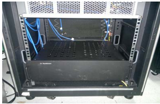
Figure 3-15 Installing the Combiner Unit
