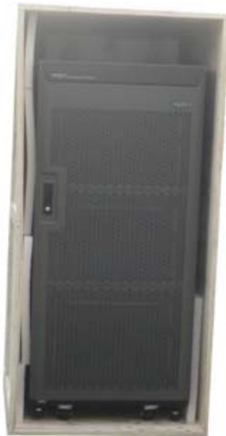
Figure 3-3 Erecting the Wooden Case
