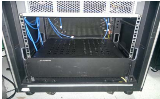
Figure 3-15 Installing the Combiner Unit
