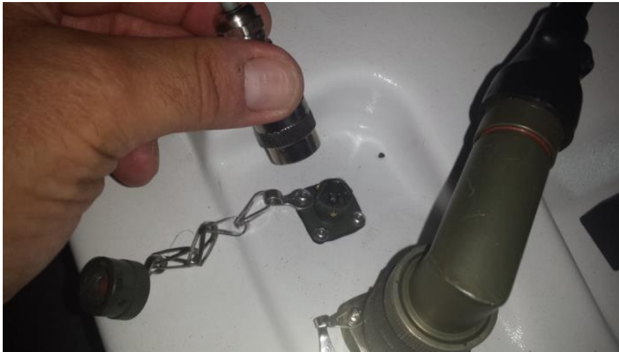
Fig. 4.9 – Connecting the second power cable to the antenna
