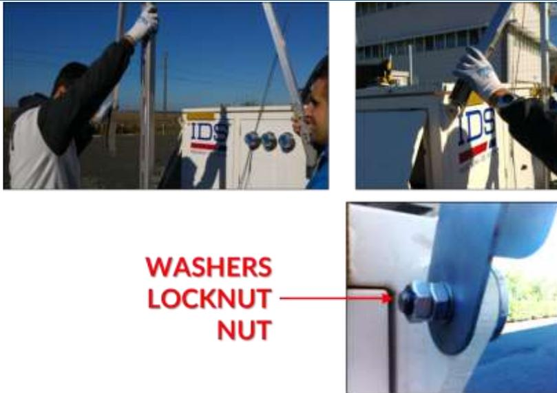
Fig. 92 – Secure the Wind Pole to the ArcSAR Supply Unit
