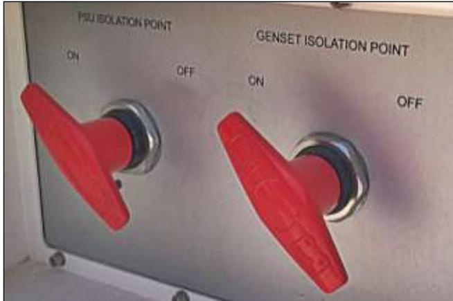
Fig. 100 – PSU and GENSET Isolation Points switch turned on
