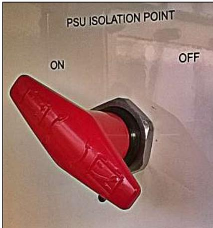
Fig. 144 – PSU Isolation Point switch turned on
