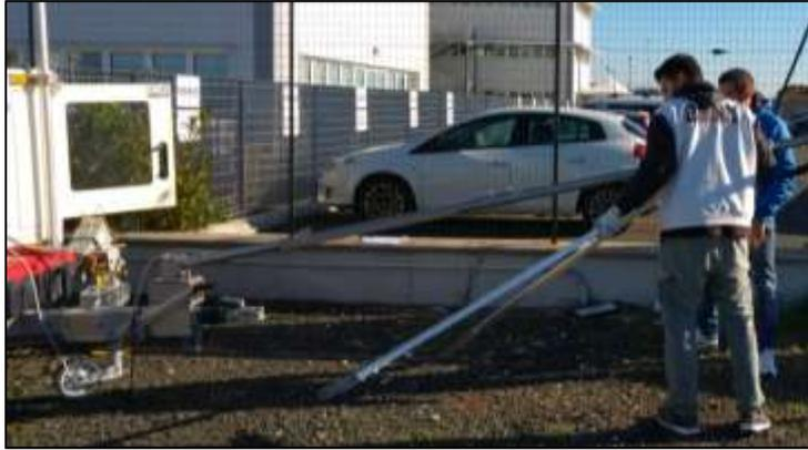
**Fig. 90 – Anchoring bars installed on the Wind Pole**
