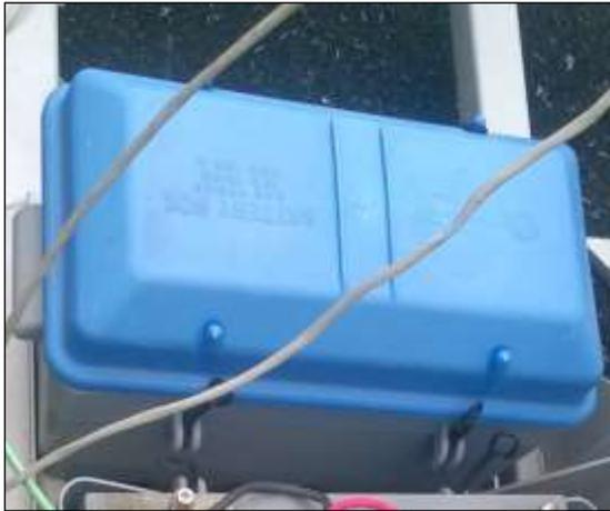
**Fig. 72 – Repeater battery with blue cover installed**
