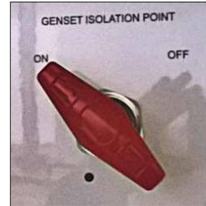
Fig. 139 – GENSET Isolation Point switch turned on
