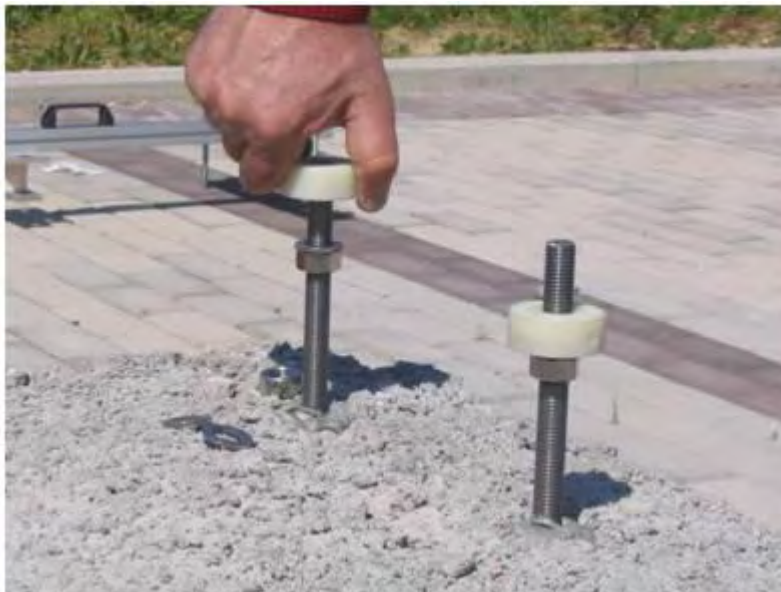
Fig. 4.11 – Mounting the base washers
