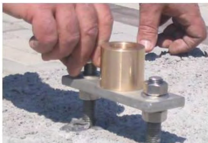
Fig. 4.14 – Mounting the fixing plate to the spherical housing
