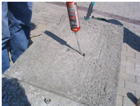
Fig. 4.10 – Resin injection operation
