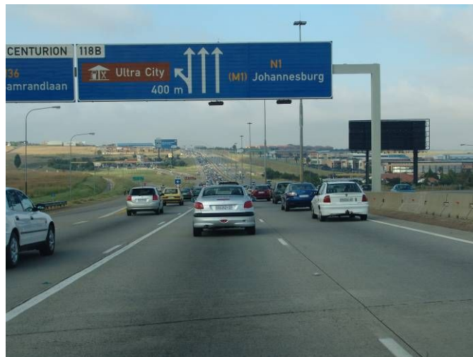
Figure 10 EVI Reader Installation: Overhead read scenario
