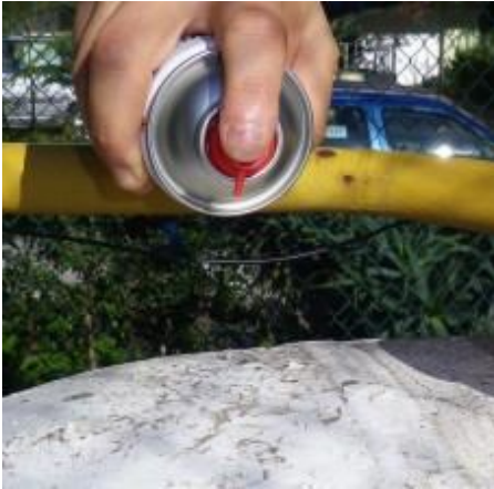
Figure 7 - Cleaning the tank surface before applying glue.
