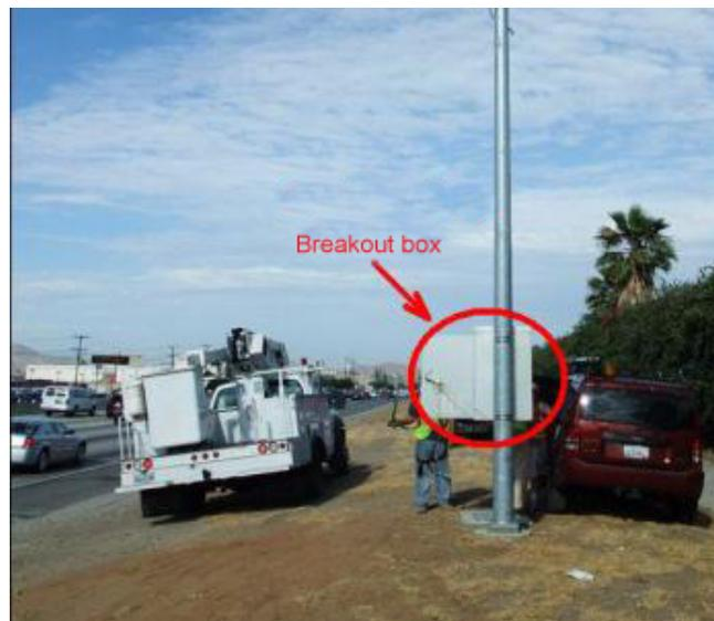
**Figure 2-3: Typical Breakout Box Installation**
