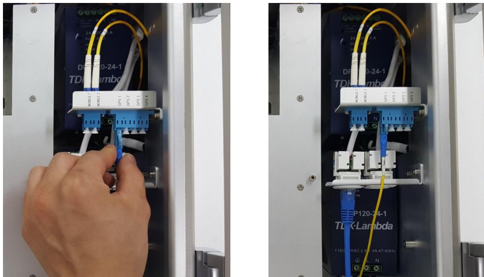
Figure 3-8 LC/UPC fiber connector connection
