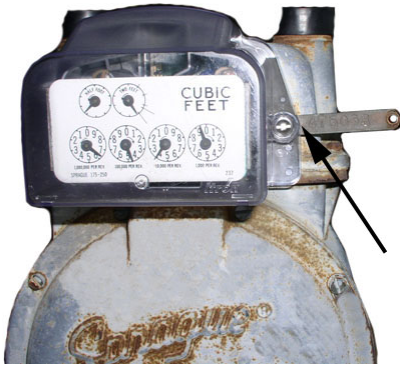
Method 2: Attach the meter tag to the 100G mounting hole
