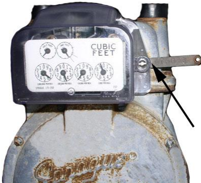
Method 2: Attach the meter tag to the 100G DLS gas ERT module mounting hole
