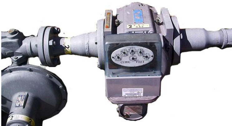
100G DLS Sensus commercial gas ERT module mounted on a GE Dresser meter with an instrument drive
