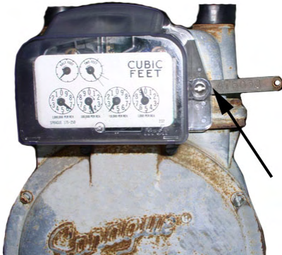
Method 2: Attach the meter tag to the 500G ERT module mounting hole
