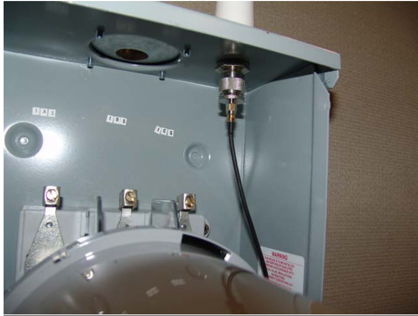
FIGURE 2 Internal connection of Laird/Antenex antenna.
