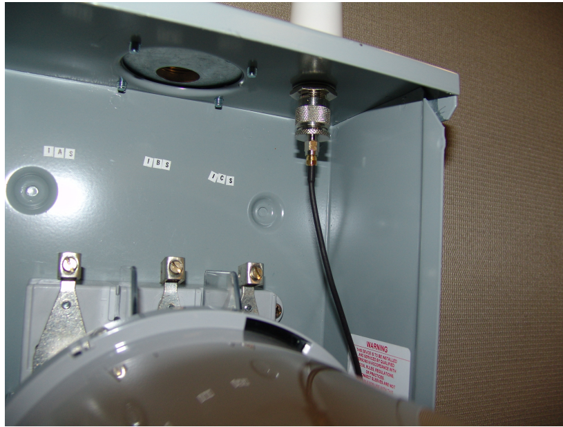
FIGURE 5 Internal connection of Laird/Antenex antenna via N-Male to SMA-Male Adapter
