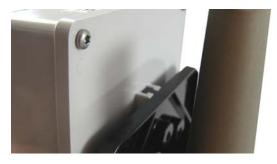
3. Install the two 1-inch remote water module mounting screws.
