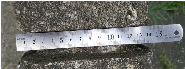
Figure 6-1 Confirmation of the wall width
