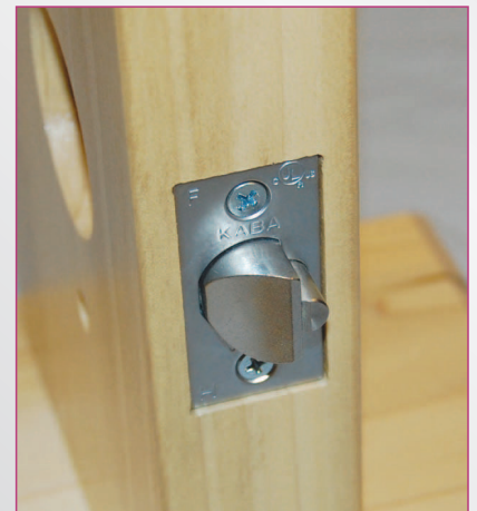
3. The first step of installation is the latch.
