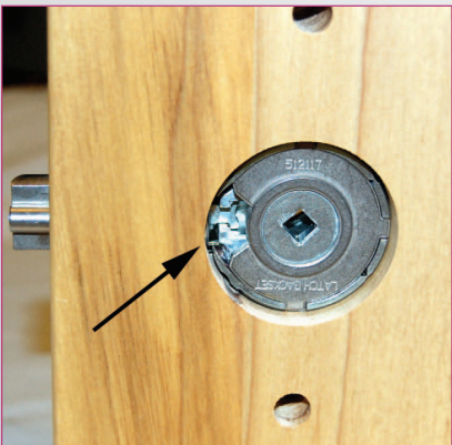
6. The latch and cylindrical unit must align properly.
