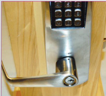
13. Turn the key 90 degrees clockwise and install the lever. Now turn it 90 degrees counterclockwise and remove the key.
