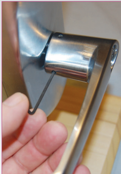
14. Don't forget to tighten the cylinder plug.
