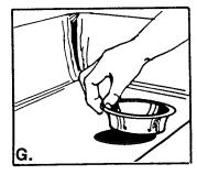
Finally, remove the old sink sleeve by pushing it up through the sink hole.
