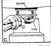
If your old disposer has a different mounting than your new one, use a pliers or adjustable wrench to remove the nuts on the mounting ring. Then remove old disposer. (Some disposers have to be removed by taking off a clamp or by twisting the disposer to remove it from its mounting. Easy to figure out.)
