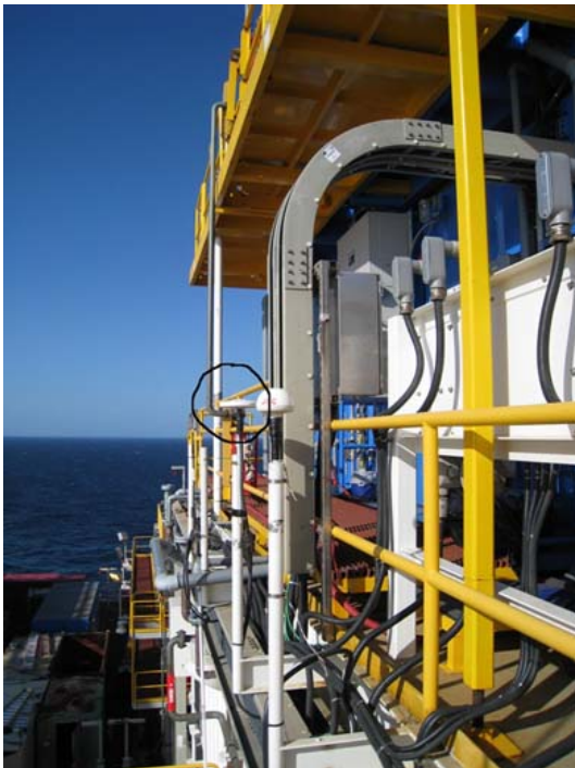
Figure 2 Bad antenna location, typically masking situation
