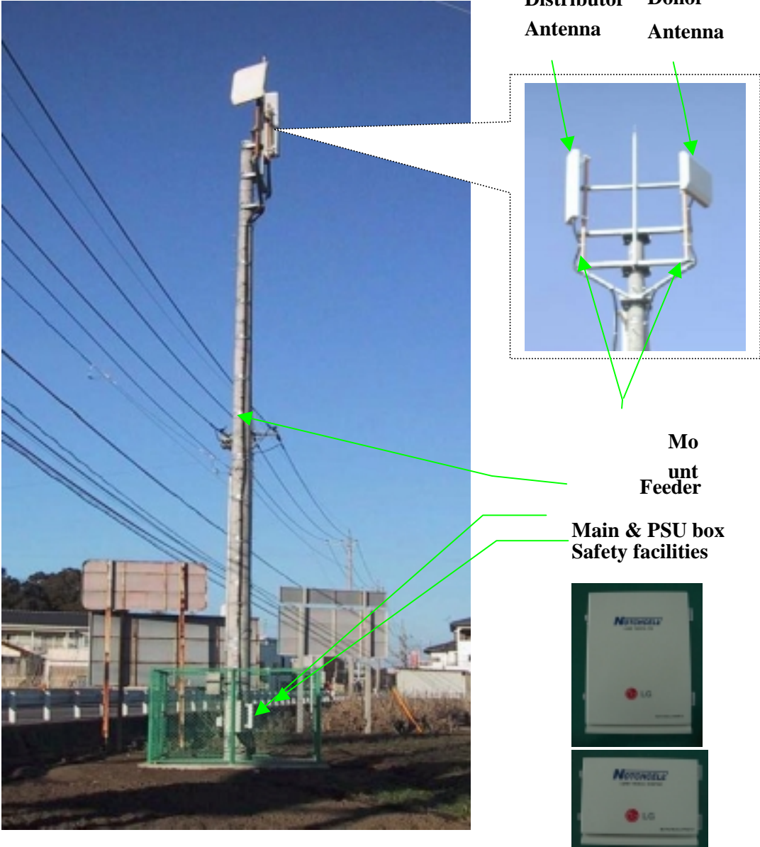
[Figure 3-1] Definition of assemblies (ex. electric pole)
