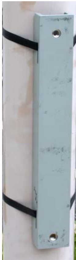
Figure 4 - 4. Strap mount pole bracket attached to pole
