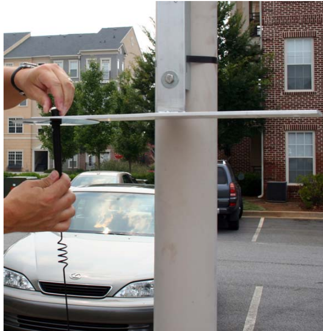
Figure 4 - 9. Connecting a LAN antenna
