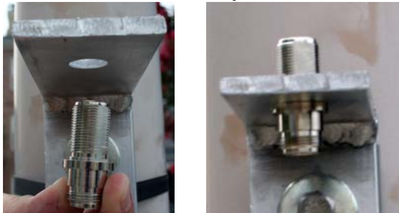
Figure 4 - 6. Attaching bulkhead connector
