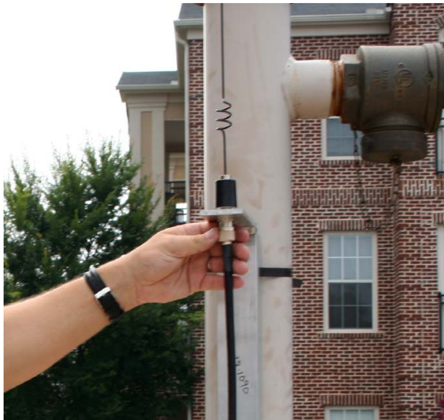
Figure 4 - 10. Attaching RF cable
